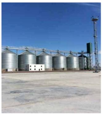
Our silos with a cylindrical body and 30° sloped roof are designed to store grains, seeds and pelletized products. Our engineering team designs its silos pursuant to various standards in order to adapt to its customers' needs including European EUROCODE and US ANSI standards.
