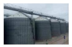
Our range of concrete base silos cover capacities ranging from 83 m<sup>3</sup> to 45,055 m<sup>3</sup> and with diameters from 4.58 m to 41.25 m.
