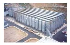
This type of silo not only brings economic savings, as no sweeping machine is necessary, but also simplifies the foundation work which considerably reduces the building costs and streamlines assembly work.
