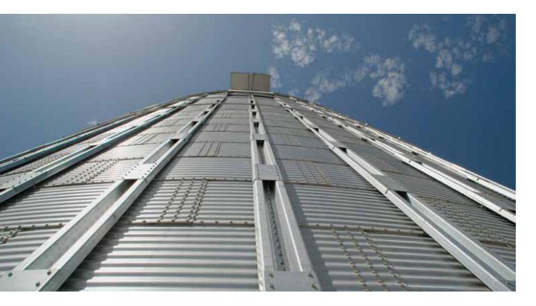
We use **high-strength steel** ranging from 350 MPa for ferrules up to 600 MPa for reinforcements, with an **innovative metal coating called ProMag.**
