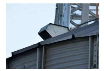
For storage plants in extreme weather zones, we have **roof protection systems** that prevent the entrance of snow into the silo through the chimneys as well as any accumulation in susceptible areas. All of our silos feature protective elements to prevent birds from entering.
